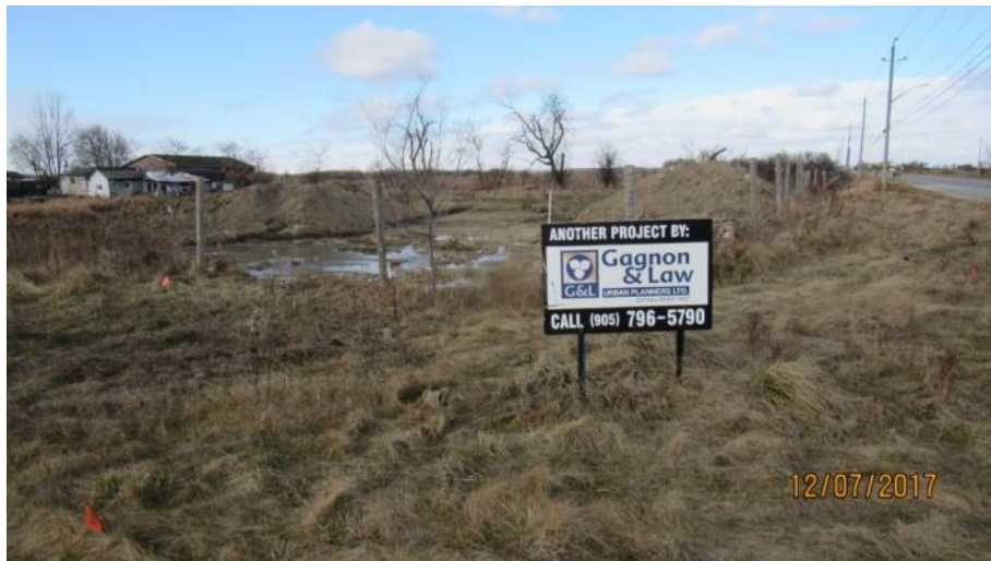
Plate 2: Northwest corner of the intersection of Airport Road and King Street, looking north.
