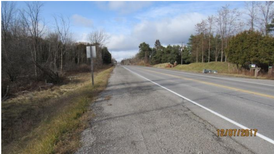
Plate 14: Gravel shoulders in the north portion of the study area, at the intersection of Airport Road and Huntsmill Drive, looking south.
