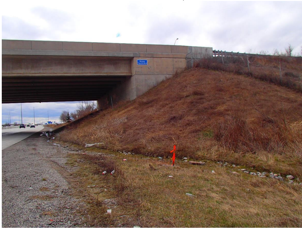
PHOTO 5: North abutment, east side
