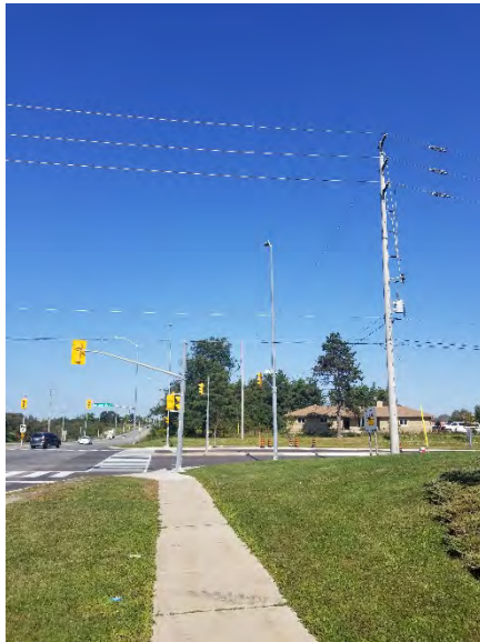
Photo 10 – A view to the north of the Site, showing an off-site property on the north and a pole mounted electrical transformer after Countryside Road.
