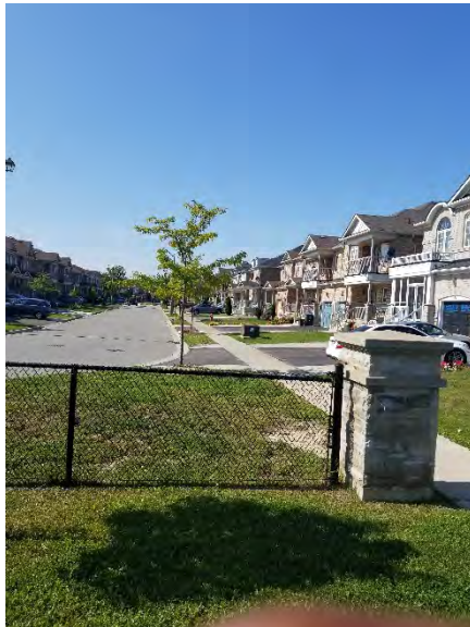
Photo 2 – View of a off-site pad-mounted electrical transformer owned by local utility company located on the west side of the Site.
