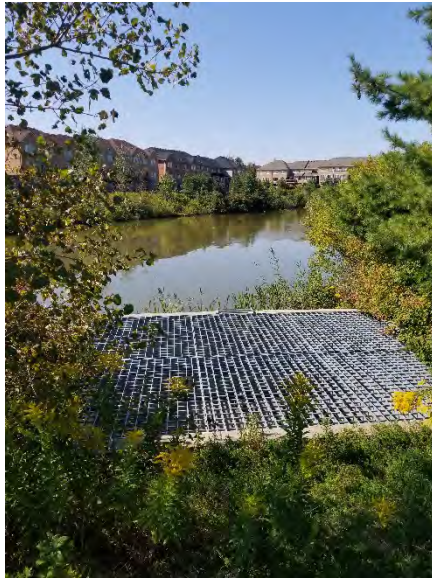
Photo 9 – A view of the southern storm water pond and surrounding properties located on the west side of the Site.
