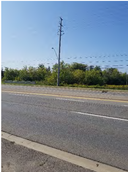
Photo 4 – A view to the west side of the Site where the northern branch of Salt Creek traverses the Site through a culvert.
