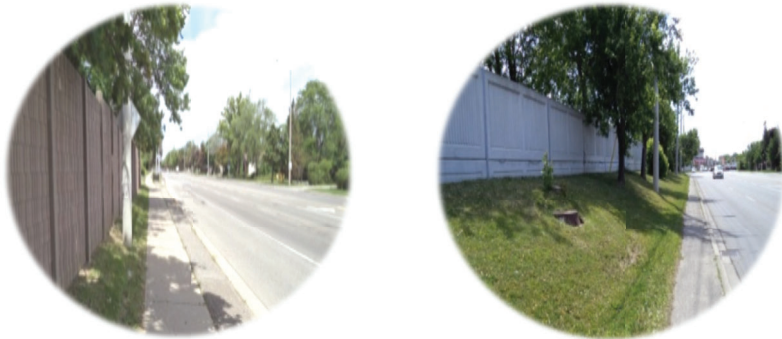
Existing Noise Walls
