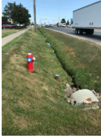
Culvert and drainage ditch located along Highway 50 in the study area.
