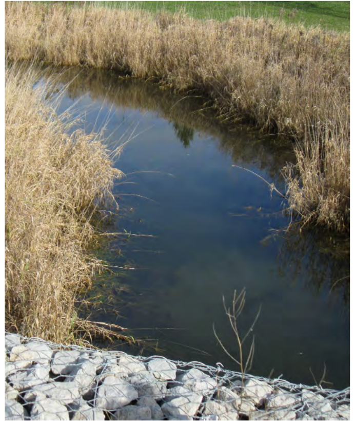
Salt Creek crossing under Airport Road
