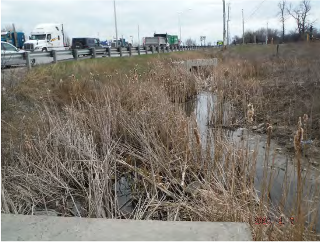
Robinson Creek southwest of RR50 and Mayfield Road looking south along west side of RR50 (April 7, 2020).
