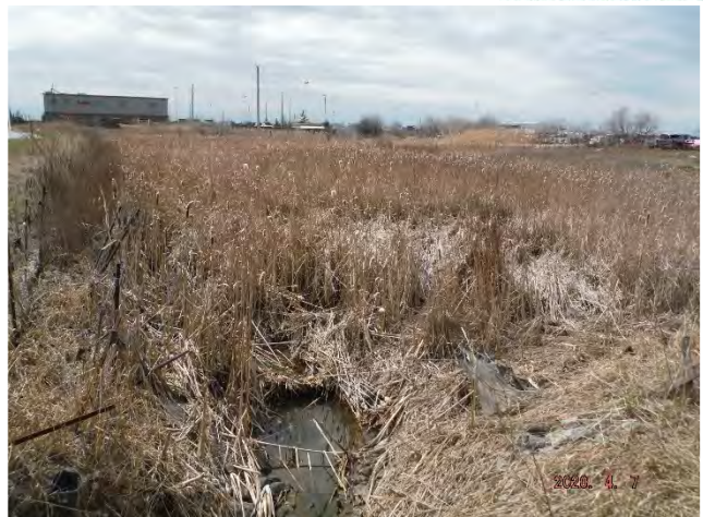
Robinson Creek northwest of RR50 and George Bolton Parkway Intersection looking northwest (April 7, 2020).
