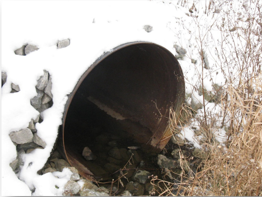
Photo 45: Culvert C16 south end
