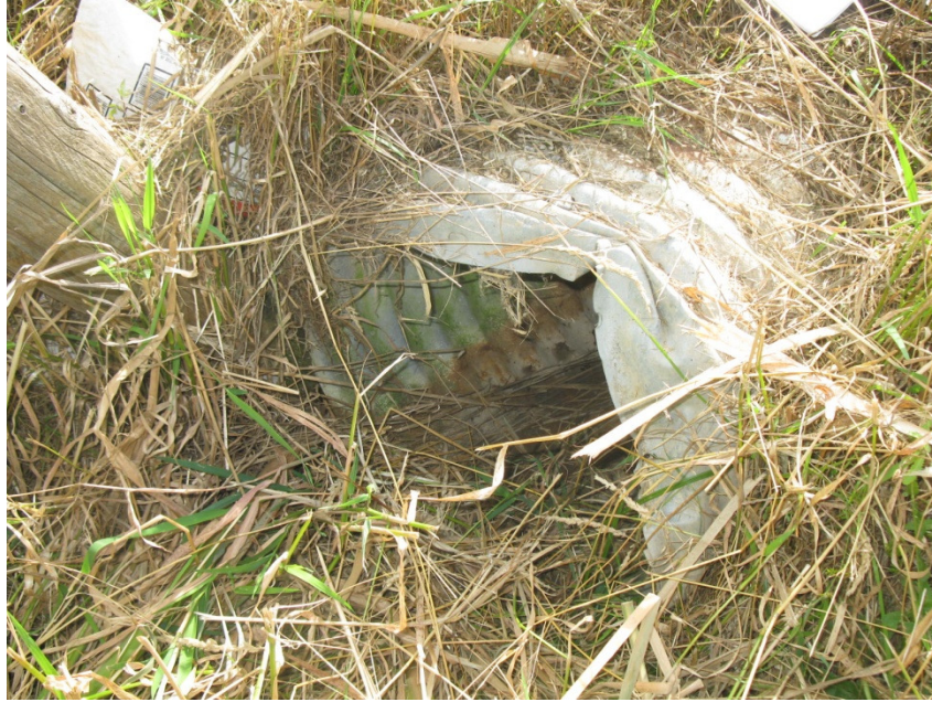
Photo 25: Culvert C10 north end
