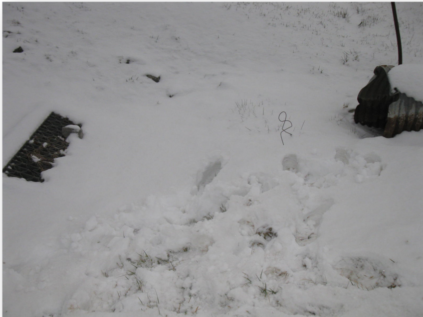
Photo 50: Ditch Inlet DI4
