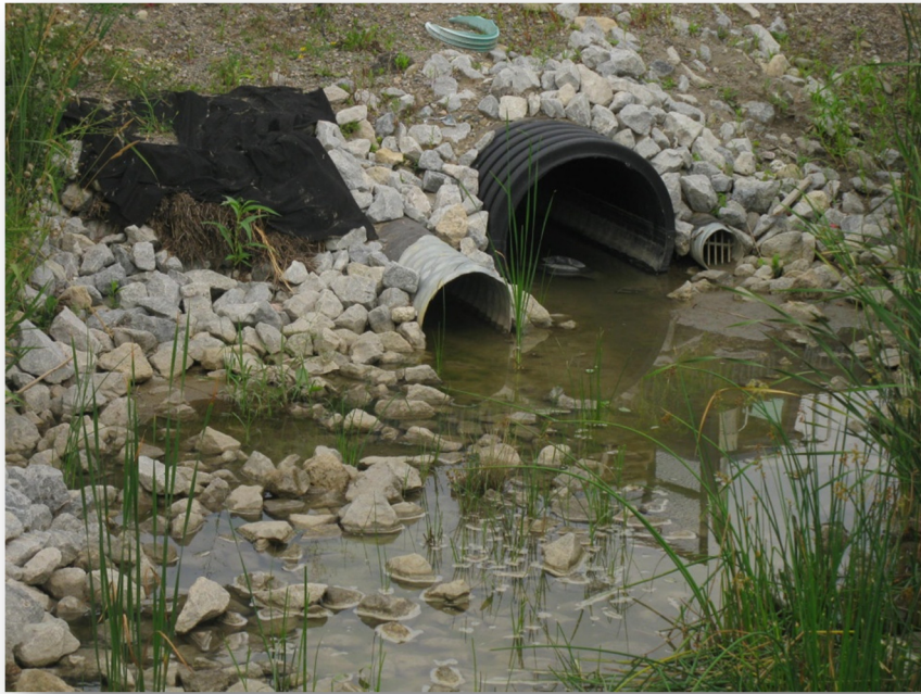
Photo 42: Culvert C15 south end
