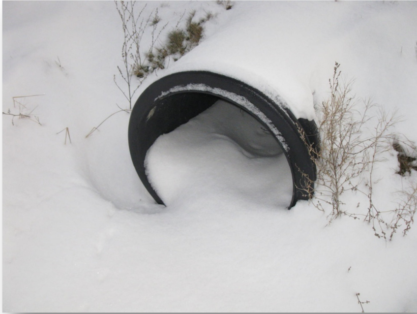
Photo 7: Culvert C4 north end
