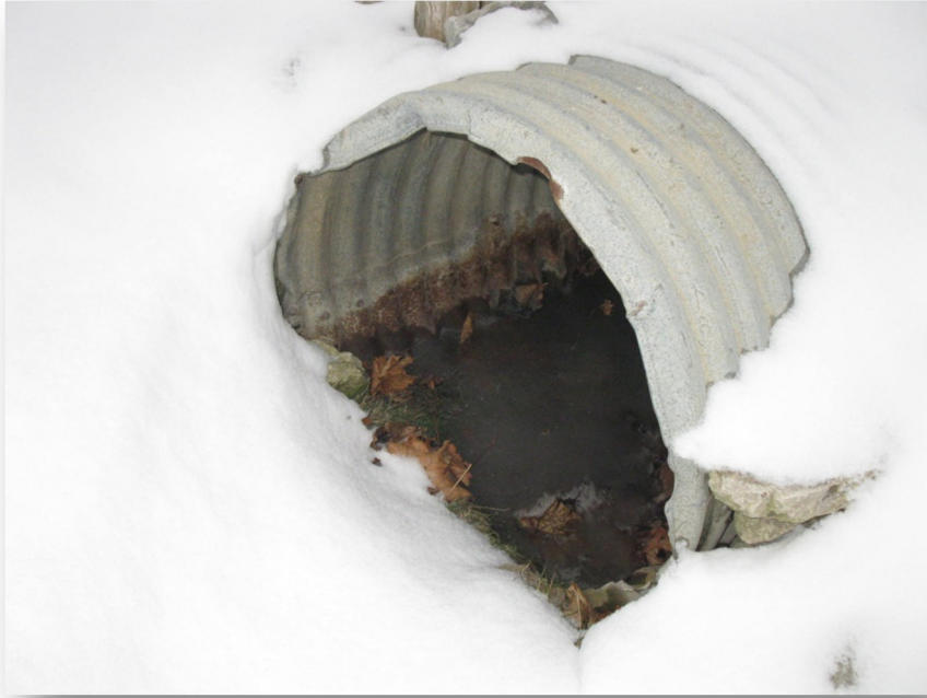
Photo 35: Culvert C13 north end
