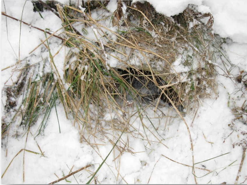
Photo 30: Culvert C11 south end
