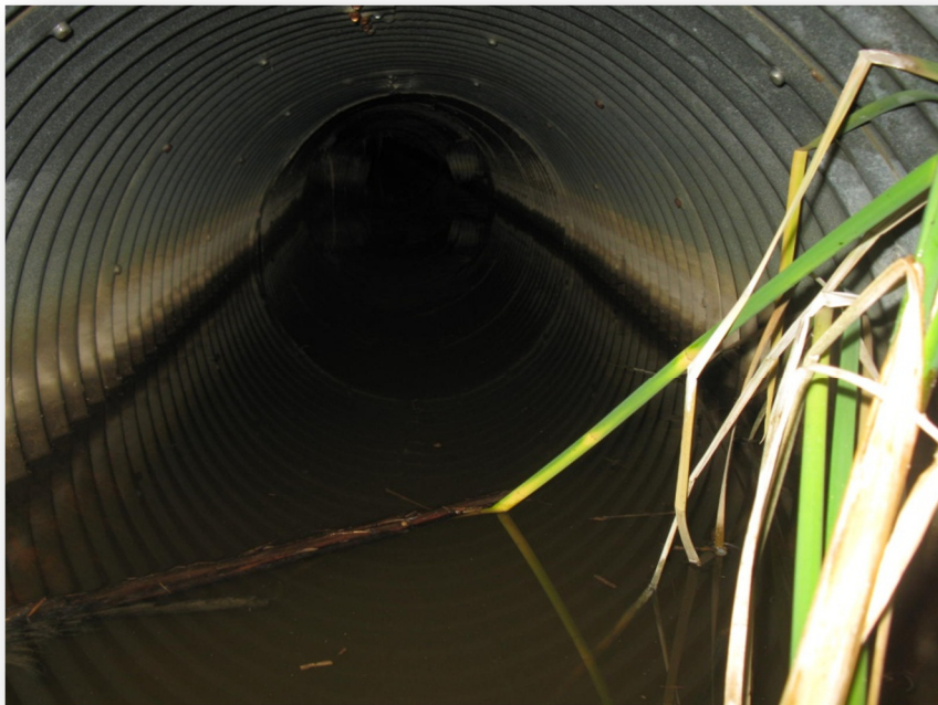
Photo 12: Culvert C6 looking inside from the north end
