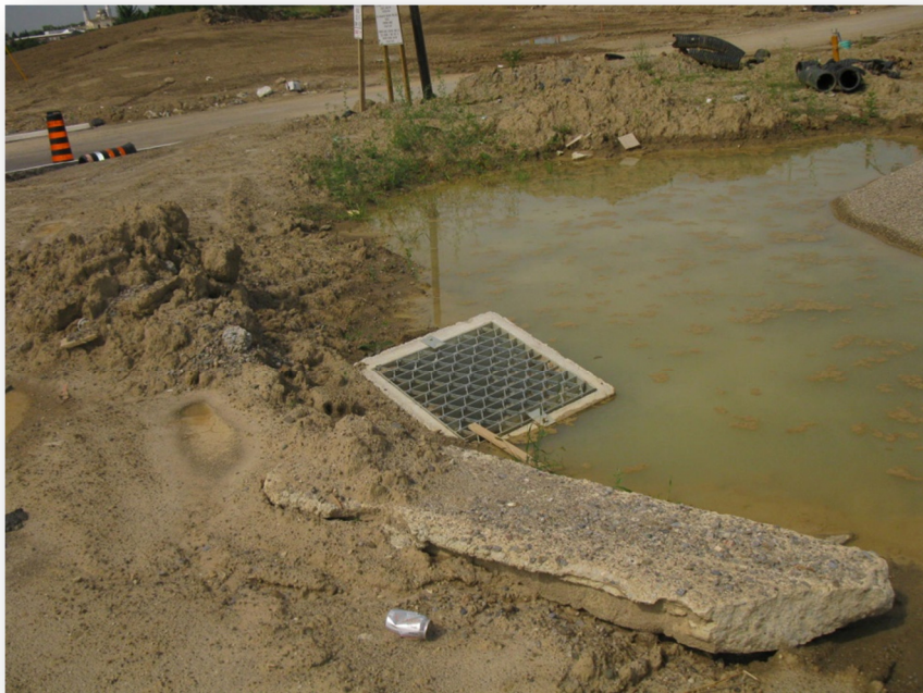
Photo 52: Ditch Inlet DI6
