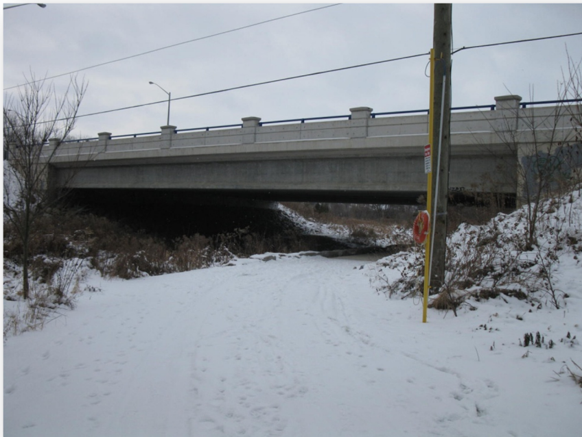
Photo 40: C14 - Etobicoke Creek Bridge south face
