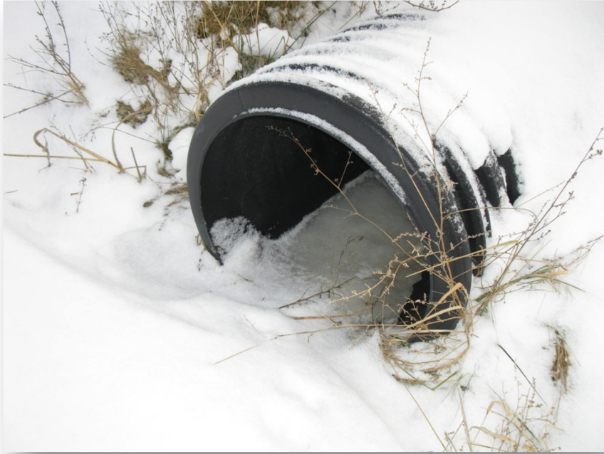
Photo 3: Culvert C2 north end
