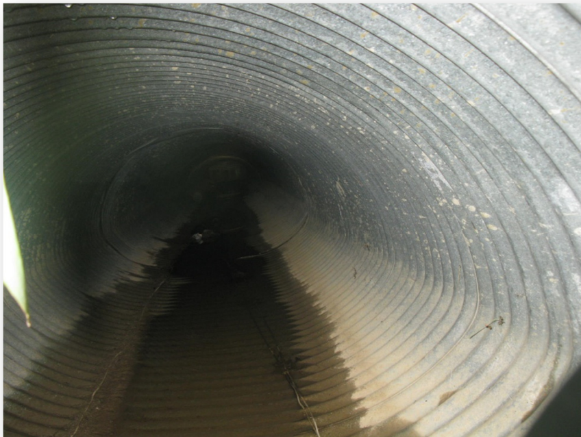
Photo 18: Culvert C8 looking inside from the north end
