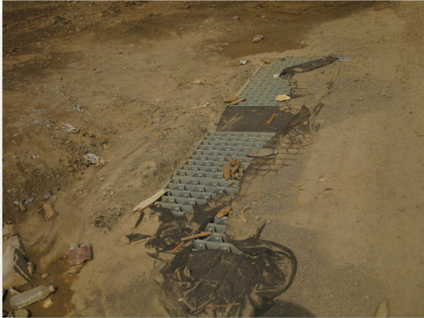
Photo 51: Twin Ditch Inlet DI5
