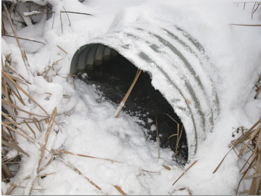
Photo 11: Culvert C6 north end
