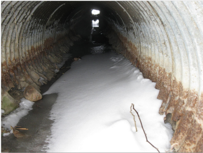
Photo 38: Culvert C13 looking inside from the south end
