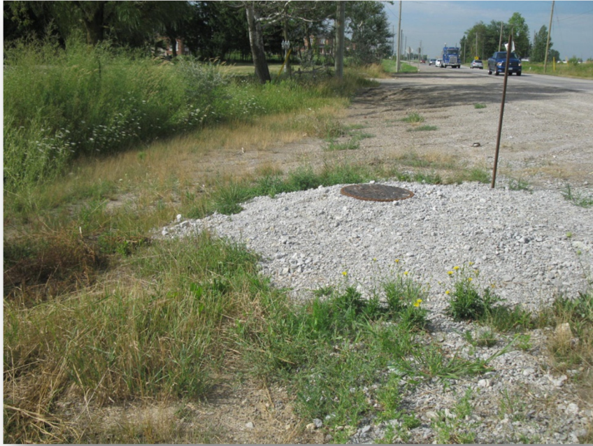
Photo 27: Culvert C10 south end – buried and storm MH exists
