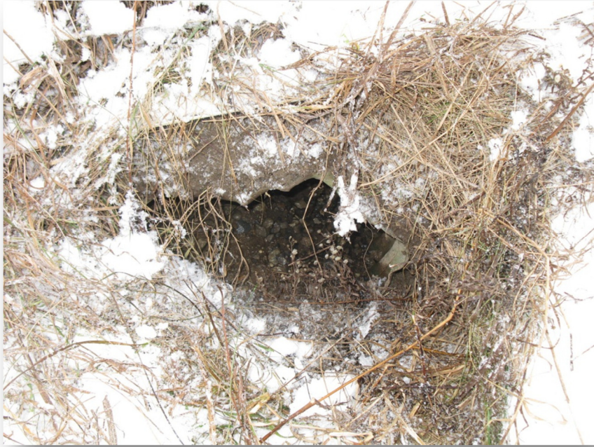
Photo 28: Culvert C11 north end
