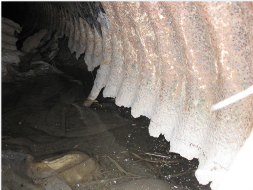
Photo 15: Culvert C7 looking inside from the north end
