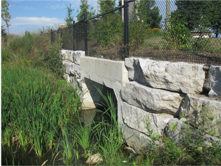
Photo 19: Culvert C8 south end
