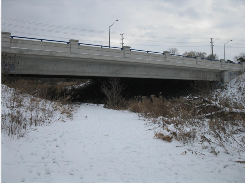
Photo 39: C14 - Etobicoke Creek Bridge north face
