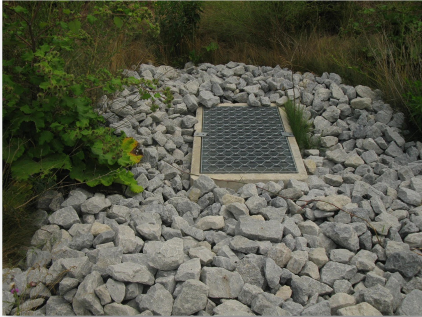
Photo 53: Ditch Inlet DI7
