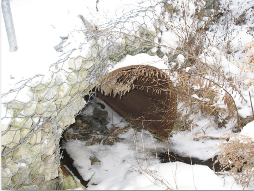
Photo 43: Culvert C16 north end
