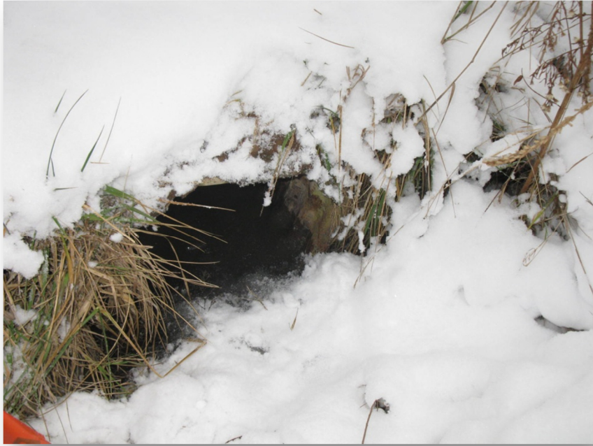
Photo 21: Culvert C9 north end
