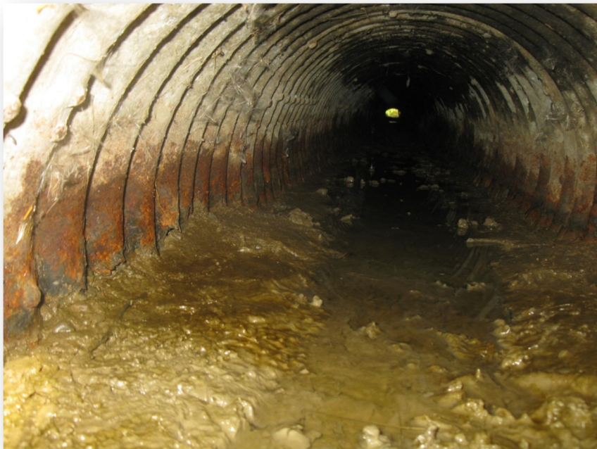
Photo 24: Culvert C9 looking inside from the south end
