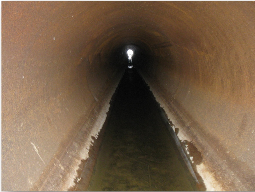
Photo 46: Culvert C16 looking inside from the south end
