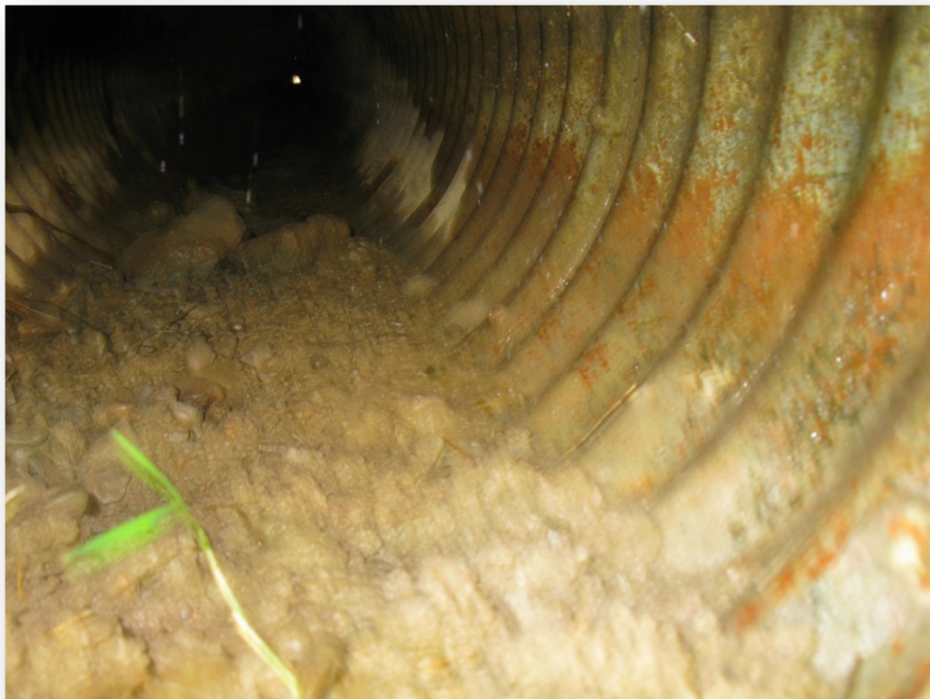
Photo 33: Culvert C12 looking inside from the north end
