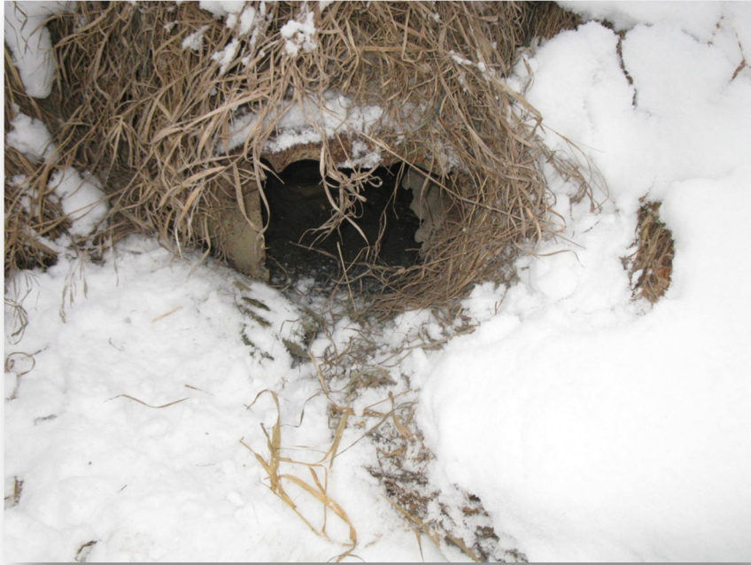
Photo 14: Culvert C7 north end
