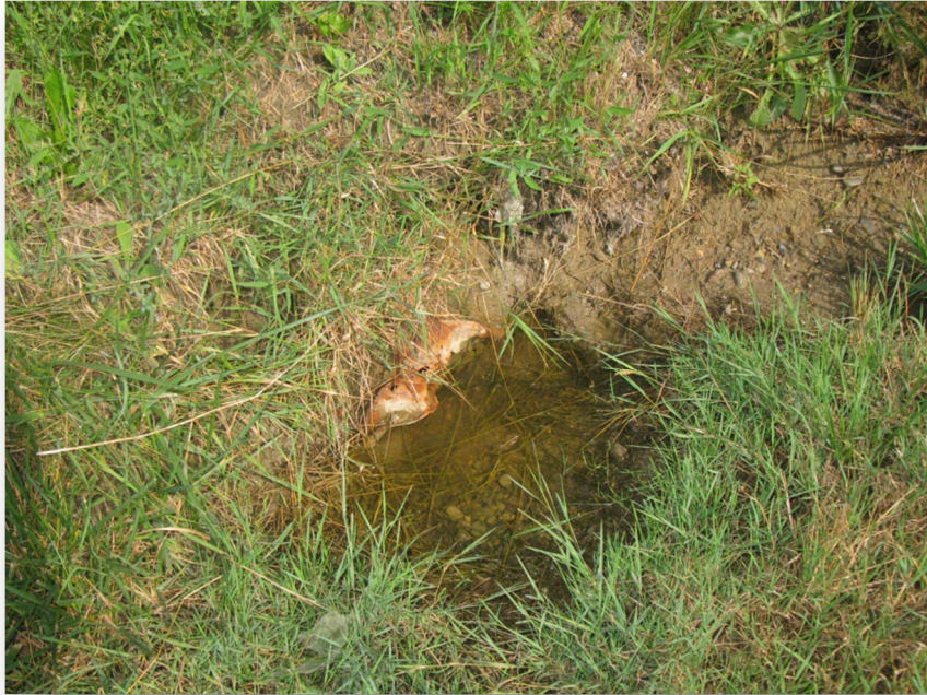
Photo 34: Culvert C12 south end
