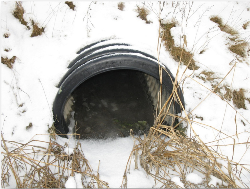
Photo 2: Culvert C1 south end
