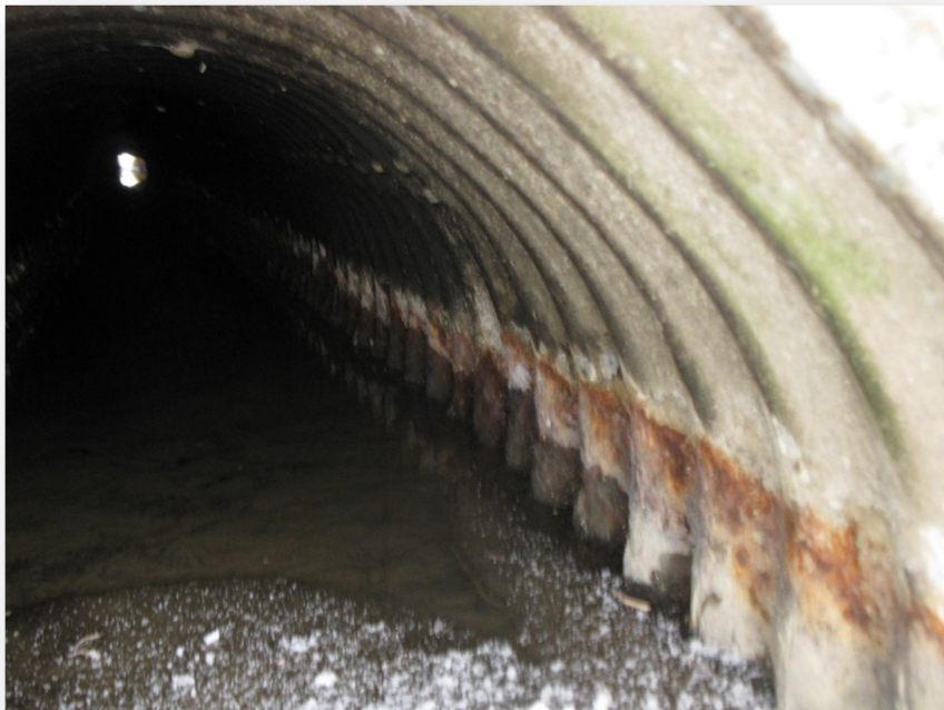
Photo 31: Culvert C11 looking inside from the south end
