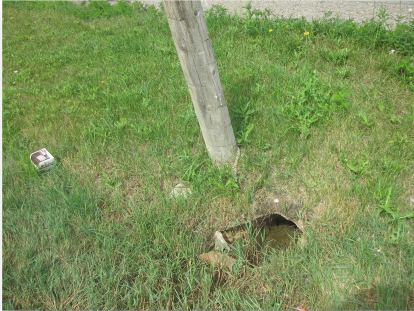
Photo 23: Culvert C9 south end
