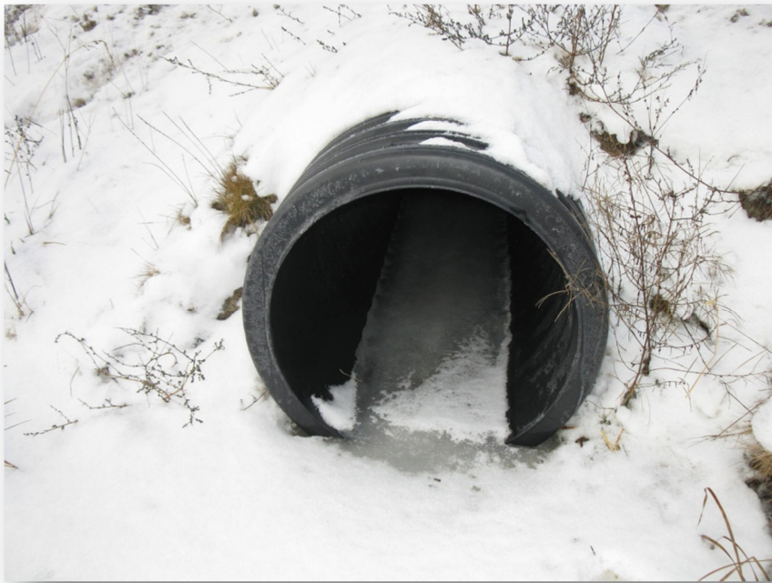
Photo 8: Culvert C4 south end
