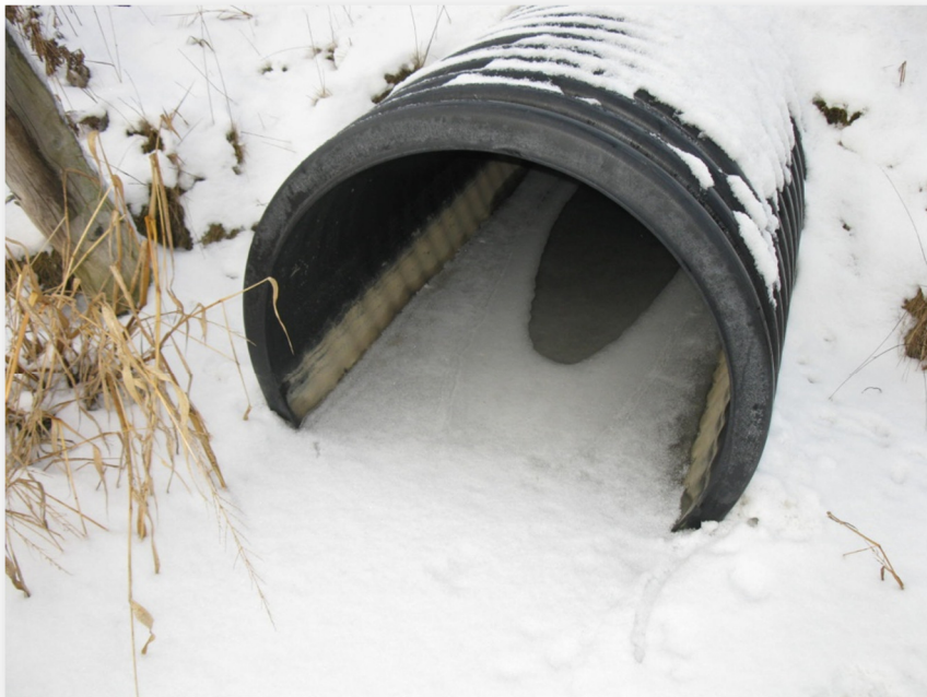
Photo 6: Culvert C3 south end
