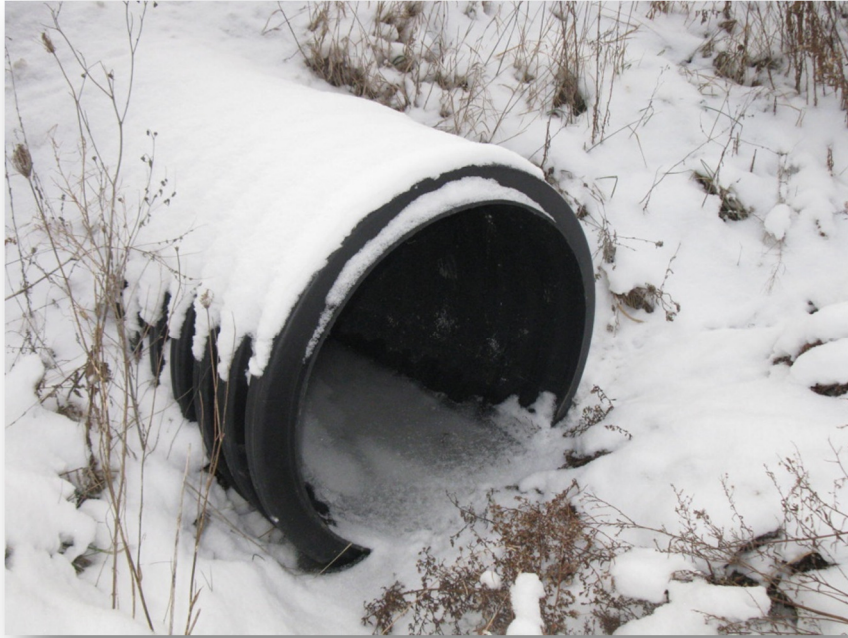
Photo 9: Culvert C5 north end
