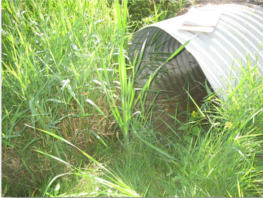
Photo 17: Culvert C8 north end
