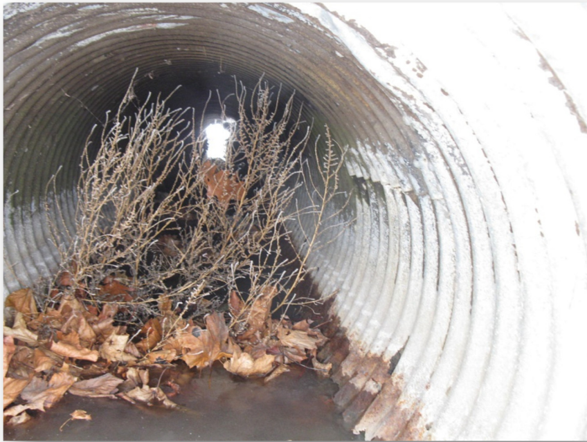
Photo 36: Culvert C13 looking inside from the north end
