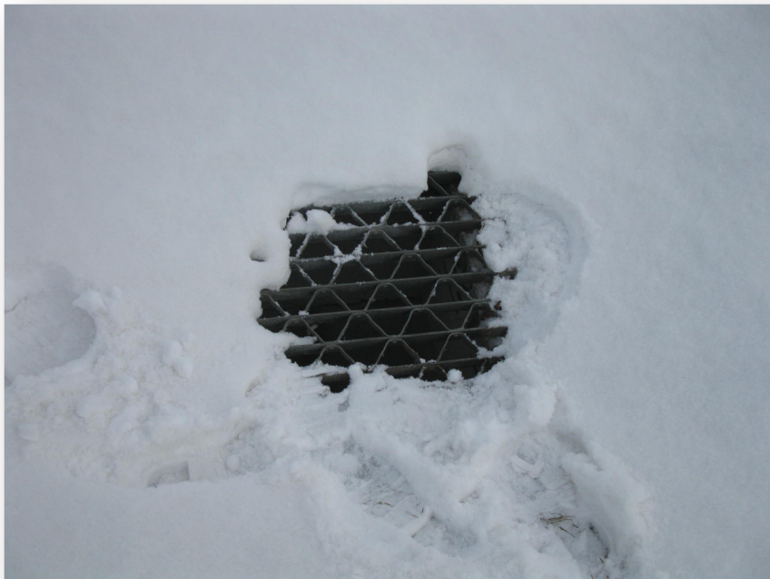
Photo 48: Ditch Inlet DI2
