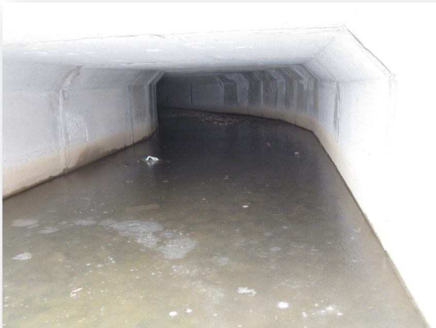
Photo 20: Culvert C8 looking inside from the south end
