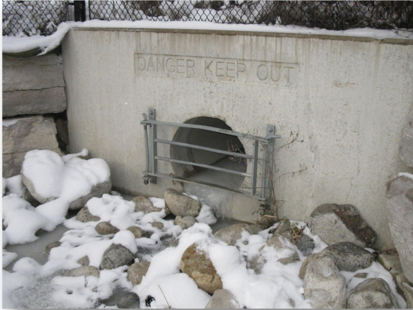
Photo 16: Culvert C7 south end
