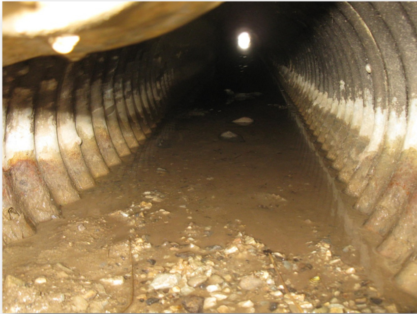
Photo 29: Culvert C11 looking inside from the north end
