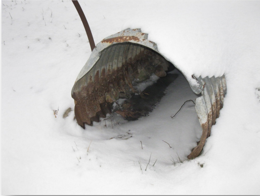
Photo 37: Culvert C13 south end
