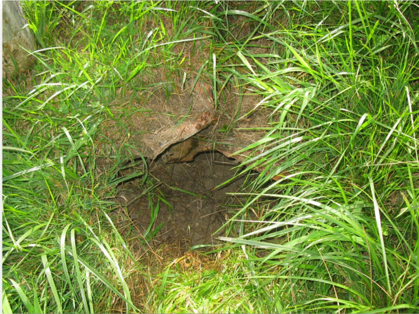
Photo 32: Culvert C12 north end
