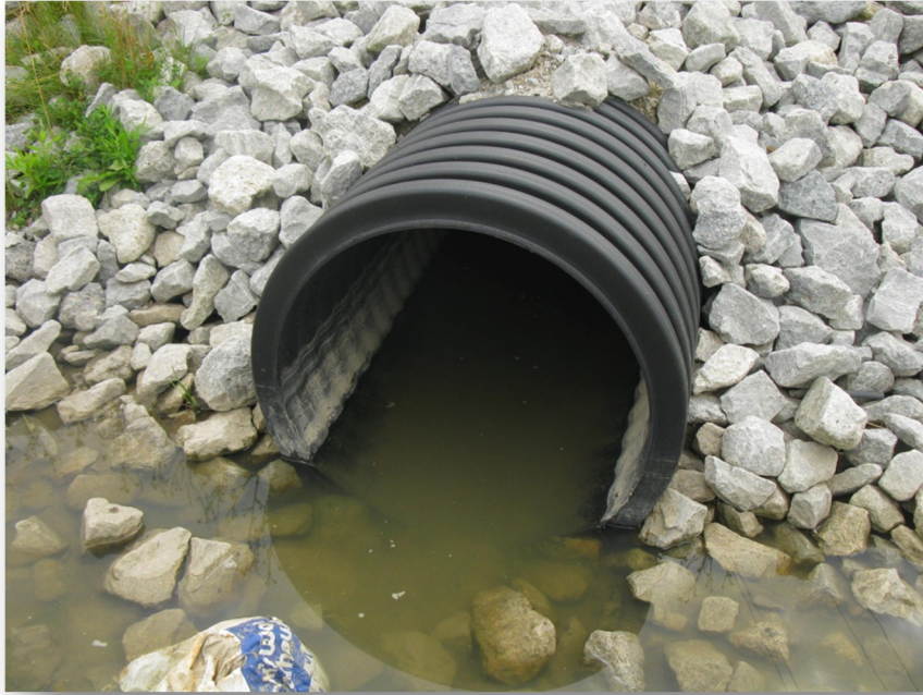
Photo 41: Culvert C15 north end
