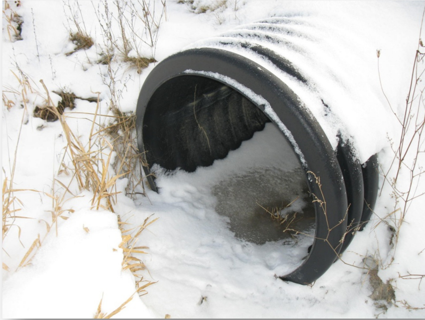
Photo 1: Culvert C1 north end
