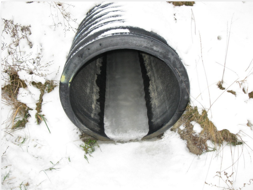
Photo 4: Culvert C2 south end
