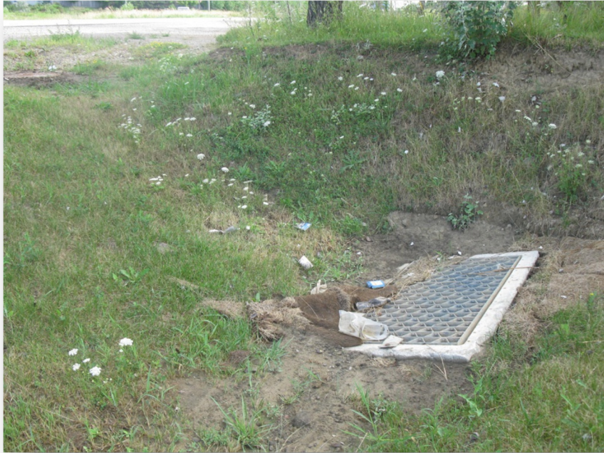
Photo 49: Ditch Inlet DI3
