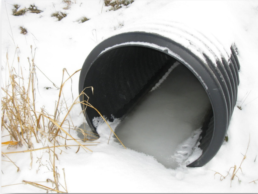
Photo 5: Culvert C3 north end
