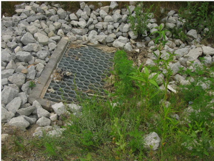
Photo 54: Ditch Inlet DI8
