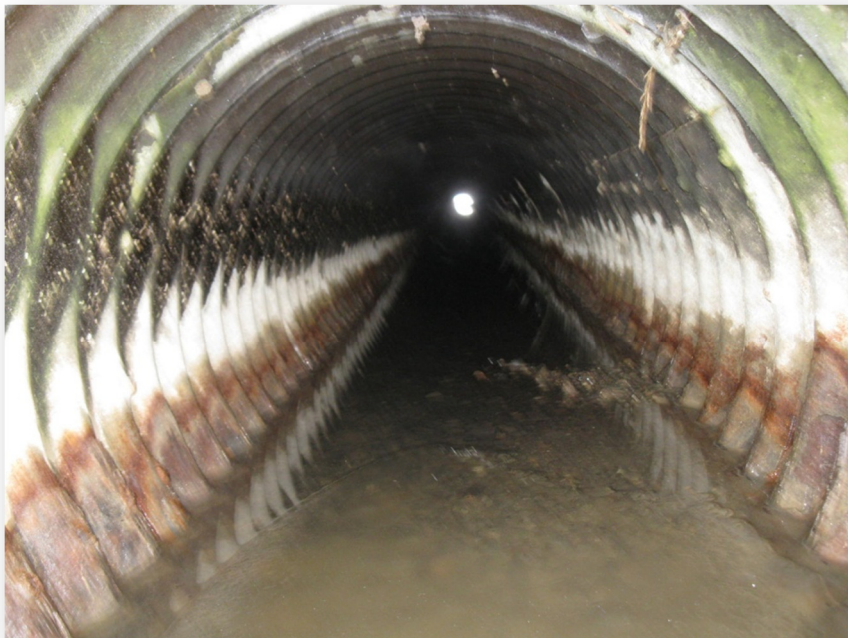
Photo 22: Culvert C9 looking inside from the north end
