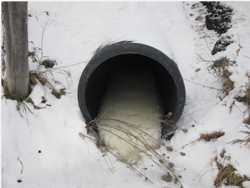
Photo 10: Culvert C5 south end
