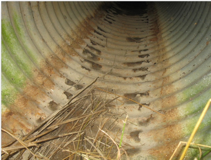
Photo 26: Culvert C10 looking inside from the north end
