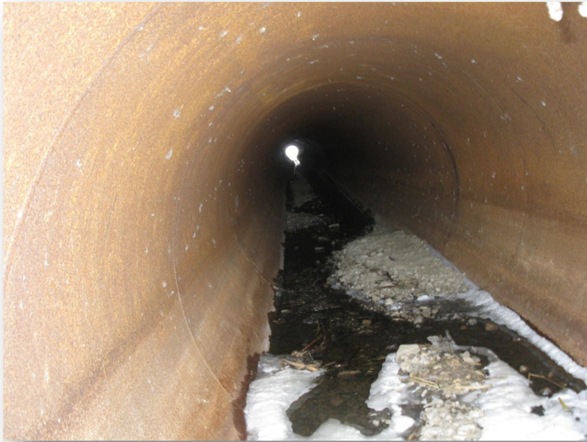
Photo 44: Culvert C16 looking inside from the north end
