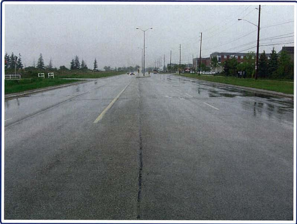
PHOTOGRAPH No.1 Sta. 13+050, Looking North.
