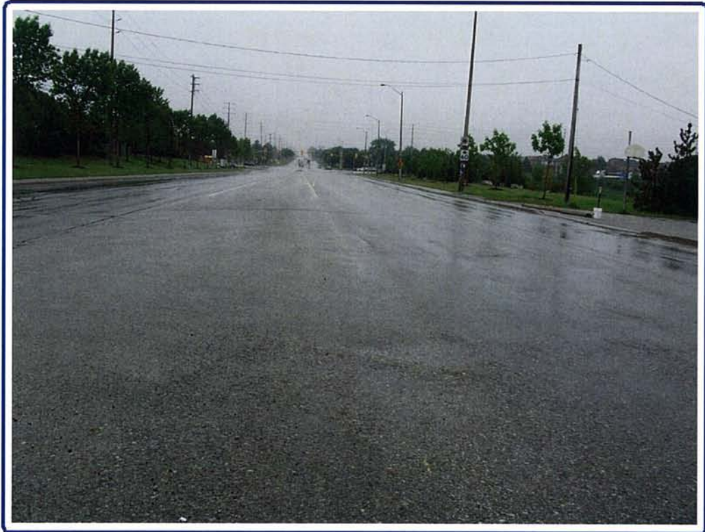
PHOTOGRAPH No.2 Sta. 10+925, Looking South.
