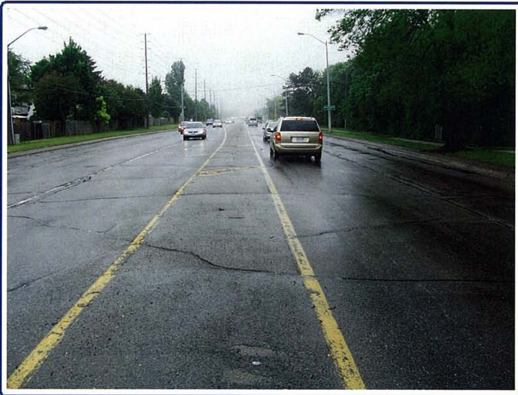
PHOTOGRAPH No.4 Sta. 8+200, Looking South.
