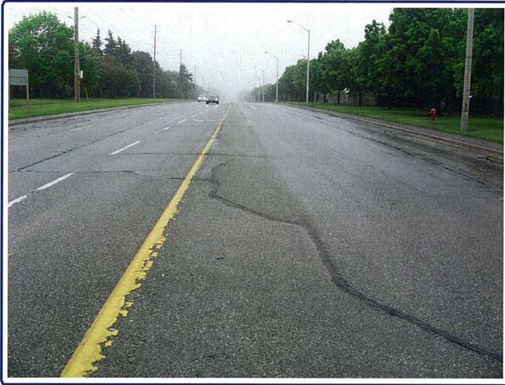
PHOTOGRAPH No.3 Sta. 9+825, Looking South.
