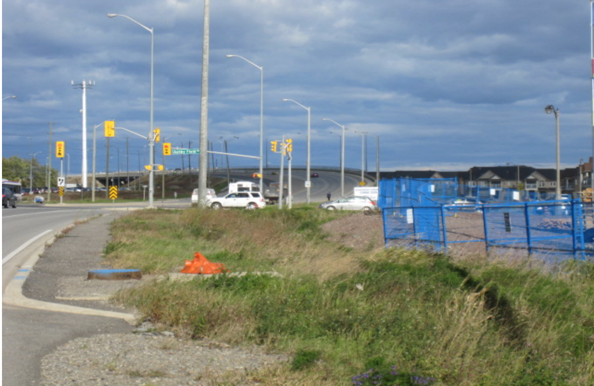
Photograph #8: A view looking east down Bovaird Drive showing the Ashby Field Road intersection and lands being prepared for development.
