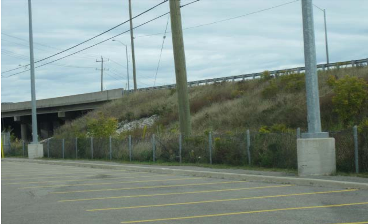
Photograph #10: A view looking east at the north side of the Bovaird Drive overpass (over the CN rail line), showing open grass slopes.
