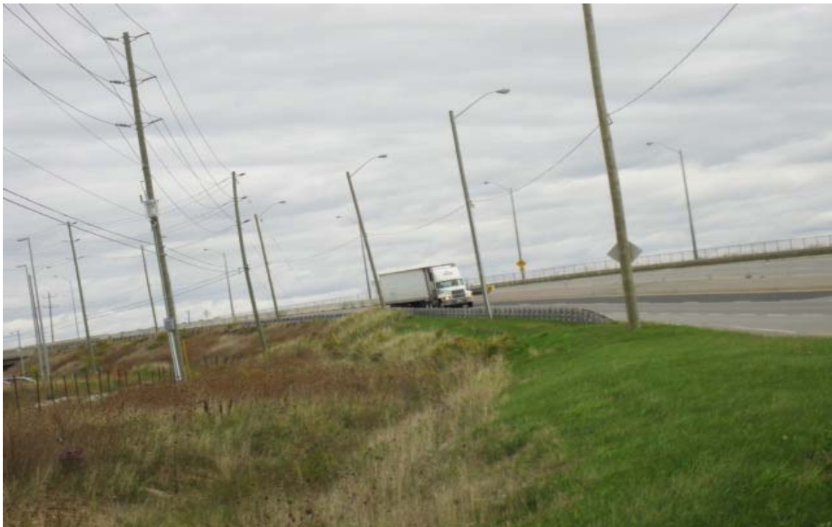
Photograph #11: A view of the grass abutment slopes on the north side of Bovaird Drive
