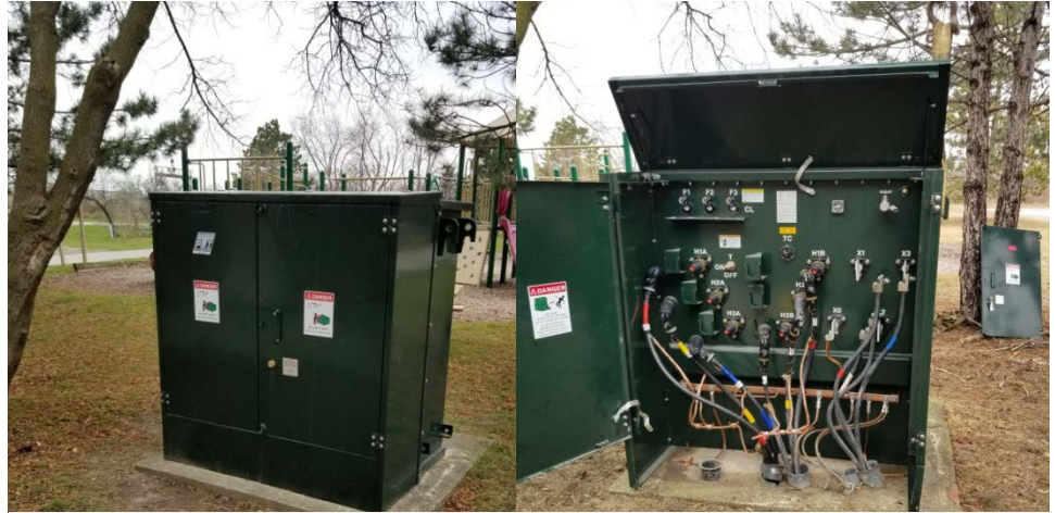
Indian Line Campground: Electrical Servicing Replacement
