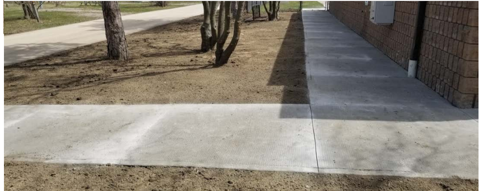
Indian Line Campground: Pool Building Waterproofing and Walkway Replacement
